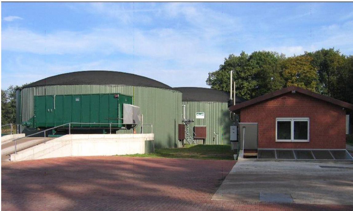
350 kW biogas plant, Germany
